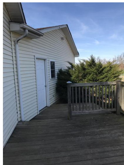
Back Deck into Garage
